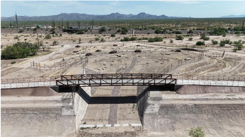
Figure 4. The newly completed wildlife ramp, with the 1-10 railroad underpass and Tortolita Mountains visible in the upper right corner. Photo by Nanda Srinivasamurthy.
