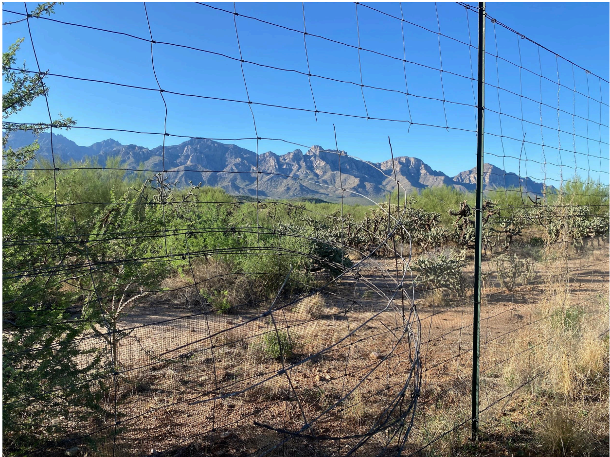
Another large opening cut into the fenceline located at 32.455001, -110.930830.
