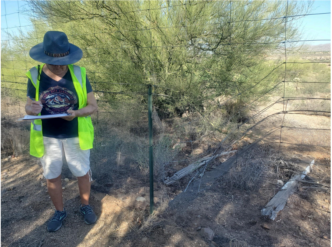
South of the wildlife bridge at 32.466672, -110.926108, close to the waste transfer station driveway. Opening large enough for people. The wire was cut deliberately but requires stepping over. Javelina tracks present here on both sides of the fence.
