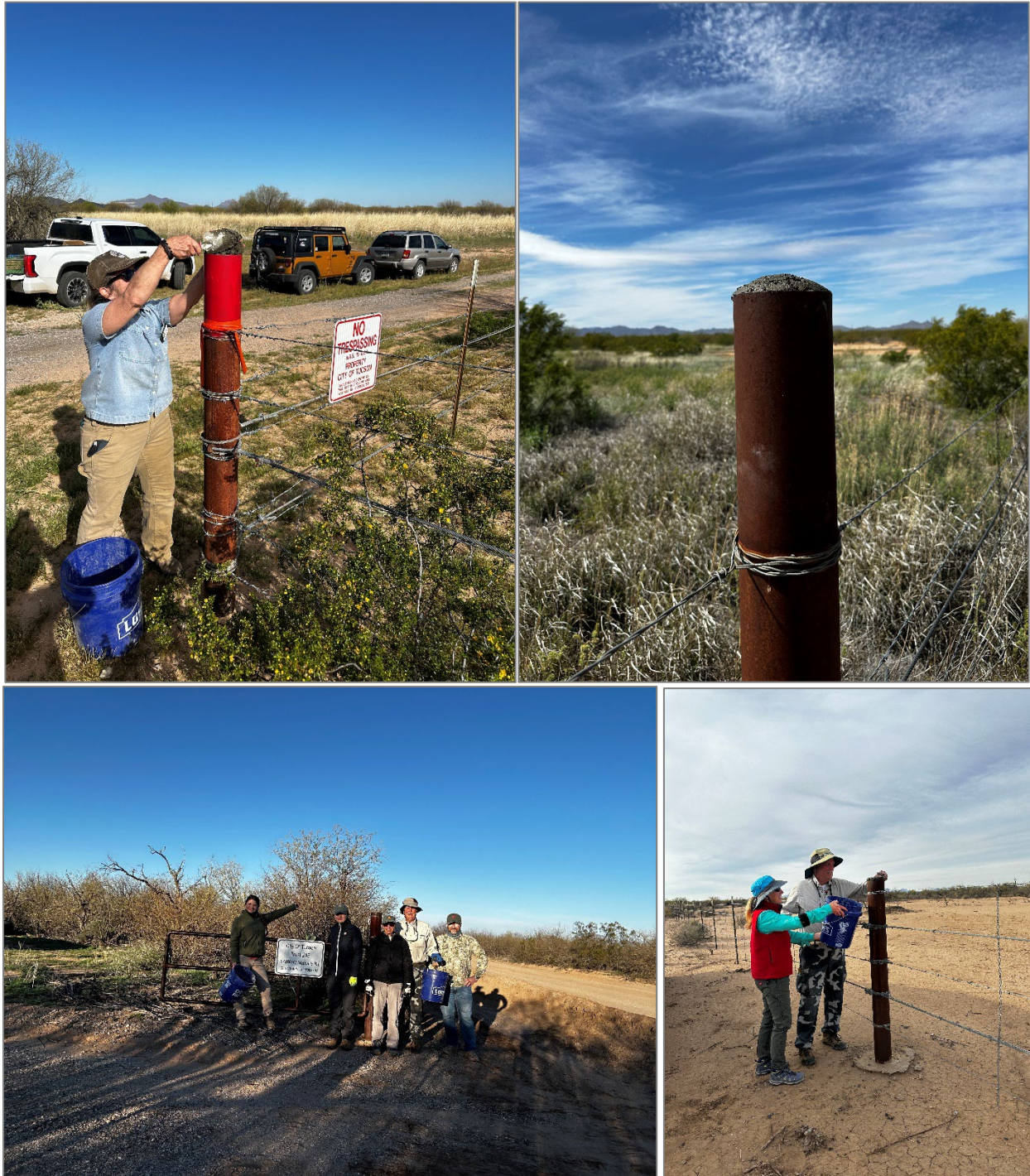
Figure 5. Volunteers capping open "death" pipes with concrete (2024). 3
