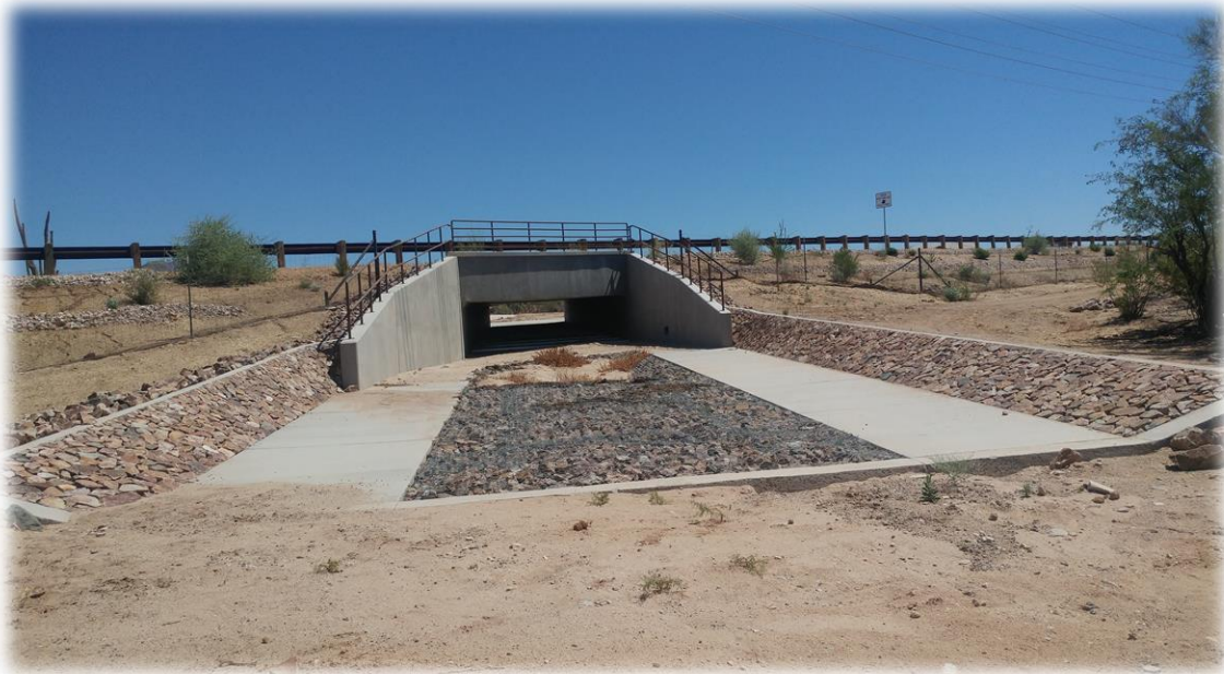
Figure 2. UP-1 viewed from the south
