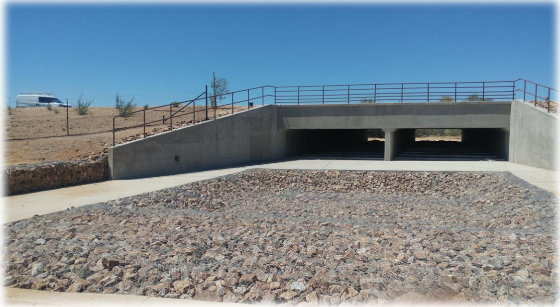
Figure 4. UP-3 viewed from the south
