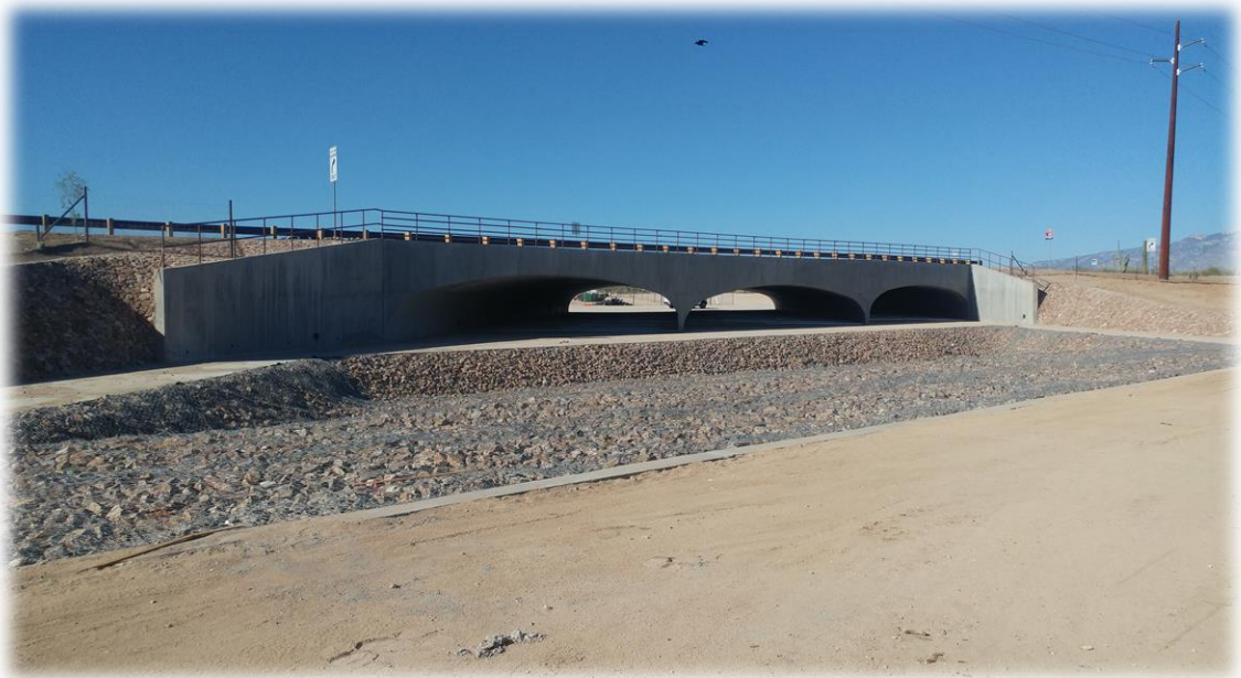
Figure 5. UP-4 viewed from the south
