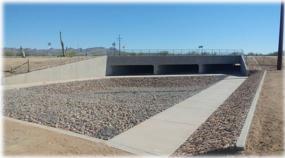
Figure 6. UP-5 viewed from the south
