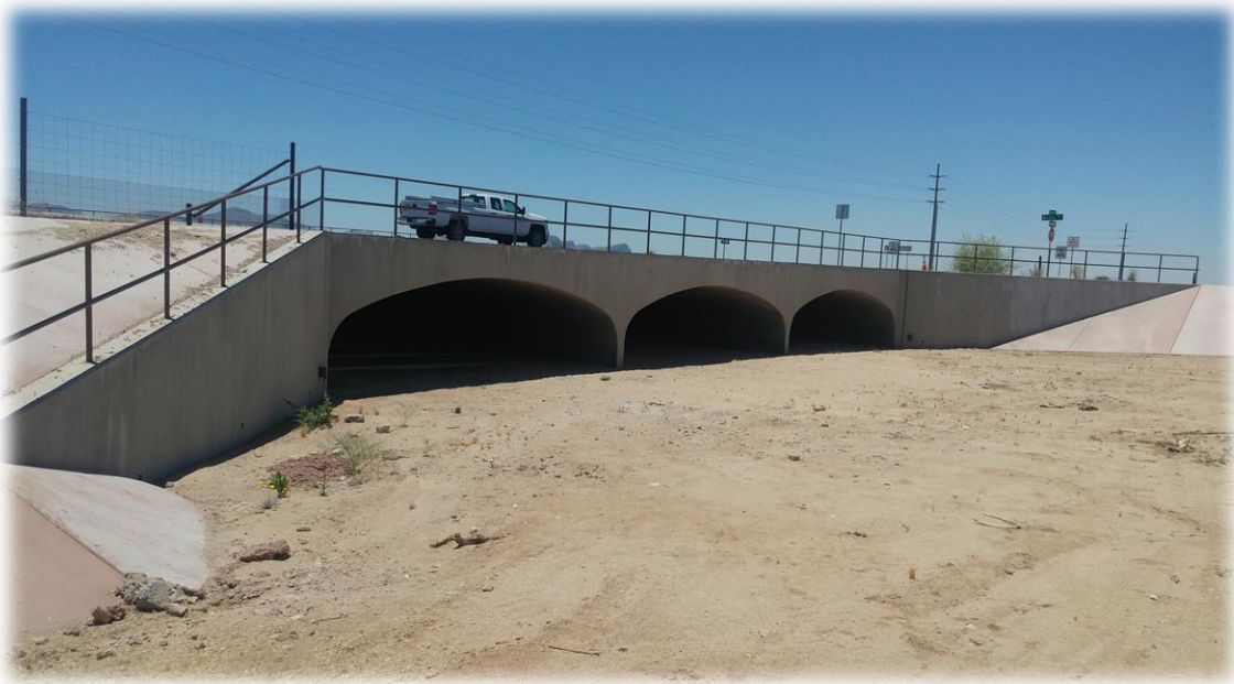
Figure 3. UP-2 viewed from the north
