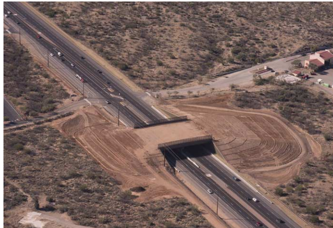
An aerial view of Pima County's first wildlife bridge providing animals a safe passage across Oracle Road. Photo courtesy Thomas Wiewandt.
