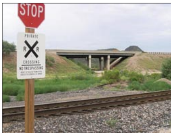
Existing underpass at I-10 and Avra Valley. Work is currently underway to preserve land on both sides of I-10 and to enhance the area to facilitate wildlife movement. Wildlife have been documented using the structure.
